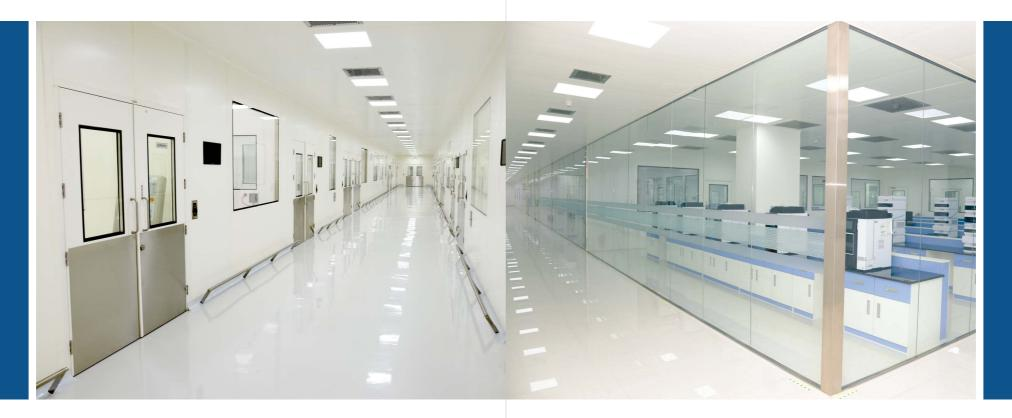
GMP modular panels are pure polyester powder coated to 60-80 microns and 15-25% gloss level with below properties
